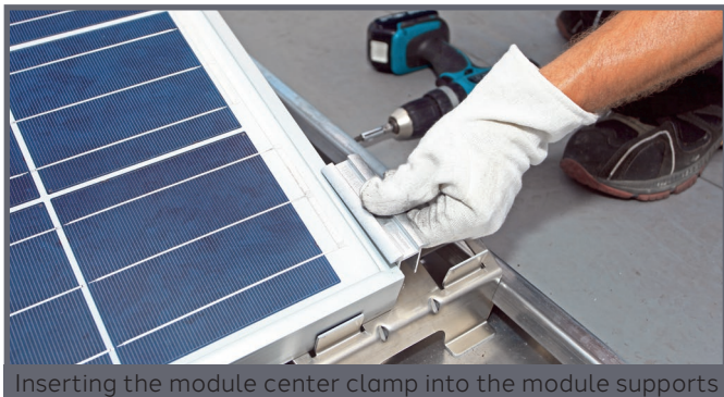
Inserting the module center clamp into the module supports
