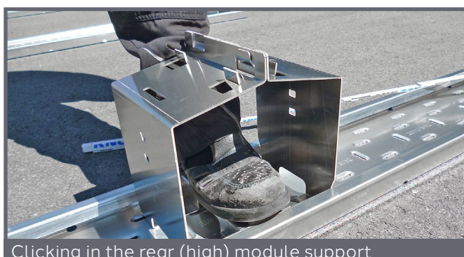
Clicking in the rear (high) module support
