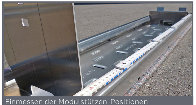
Positioning the supports
