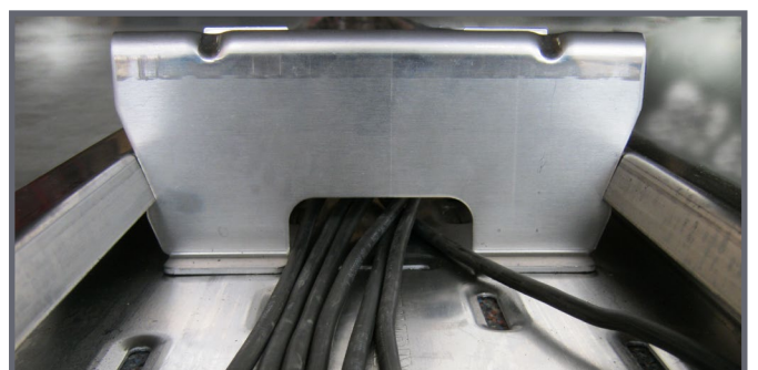
Module rail also functions as a cable tray
