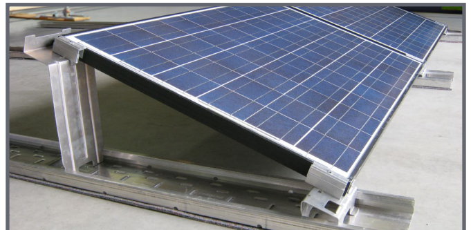
Fully assembled first row of modules
