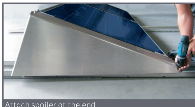
Wind deflectors fixed to floor rail
