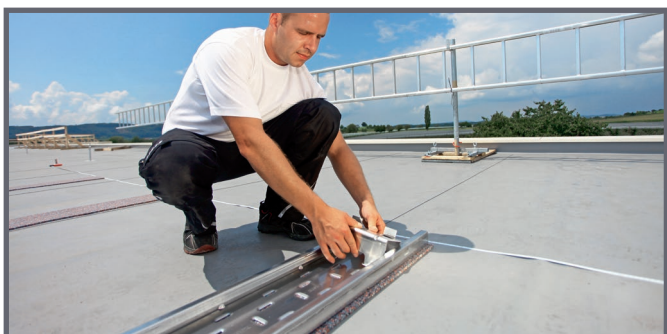
Inserting the front (short) module support
