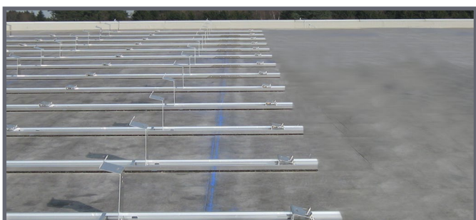
Fully assembled module supports for the first row of modules
