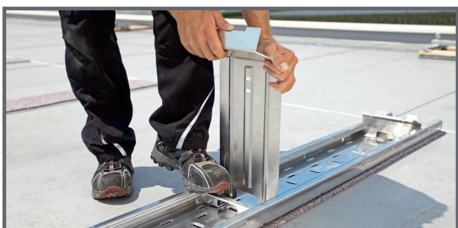
Clicking in the upper (high) module support
