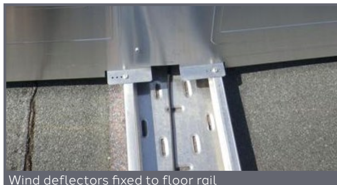
Screw the top and bottom wind deflectors together.
