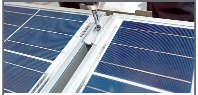
Tightening the clamps
