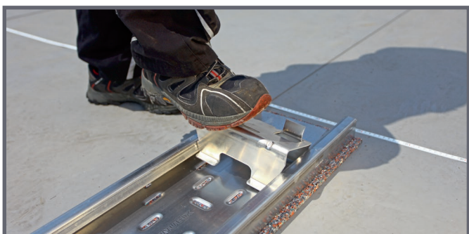
Clicking in the front module support
