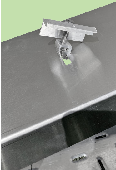
Insert the Duraklick end clamps, the nose of the clamp foot points upwards.
