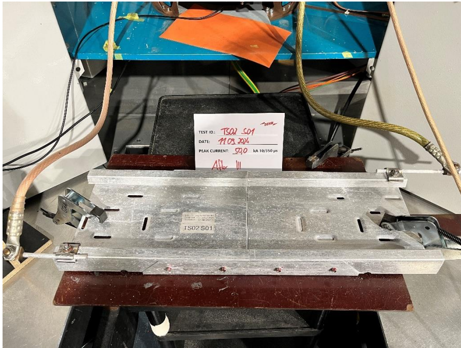
Figure 13: Test sample TS02 S01 after test with 3x 50 kA (10/350 µs).
