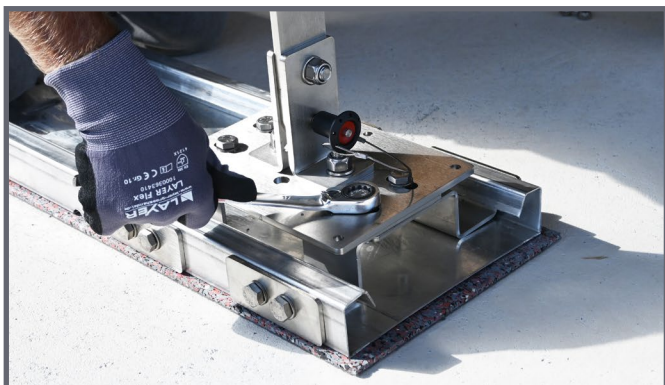
Position and Fasten Base Plate
