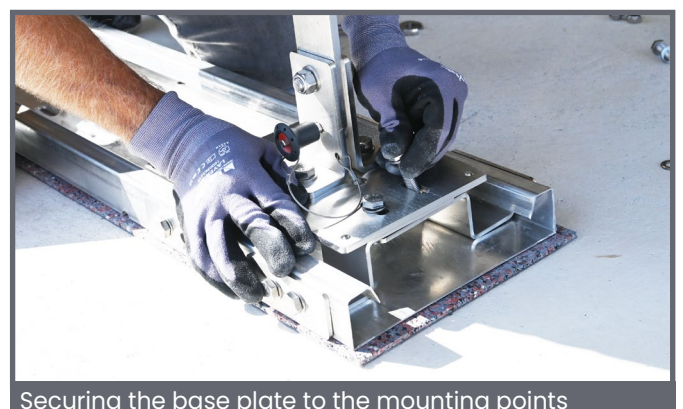
Fasten EAP to base plate
