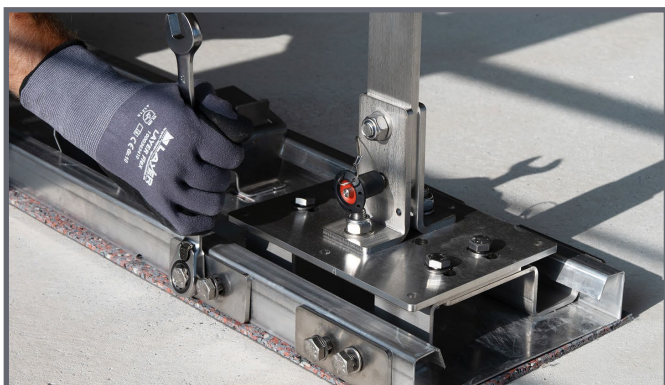
Secure screws from the side
