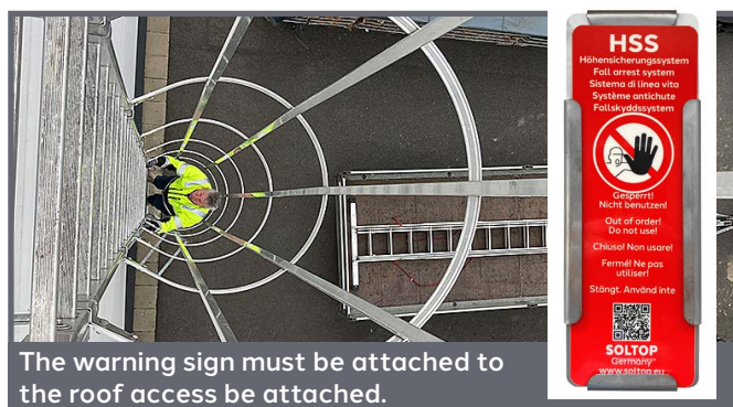
Attaching the type plate to each entrance
