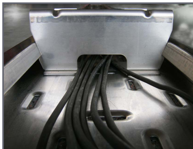
Module rail also functions as a cable tray
