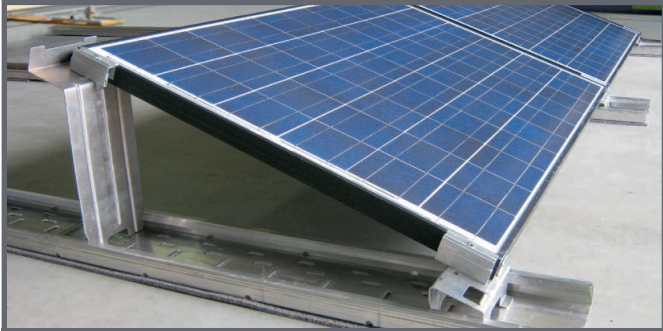
Fully assembled first row of modules
