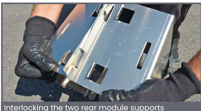
Clicking in the rear (high) module support
