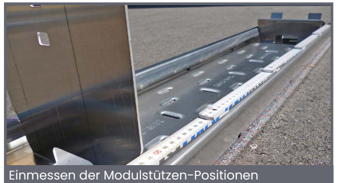
Positioning the supports
