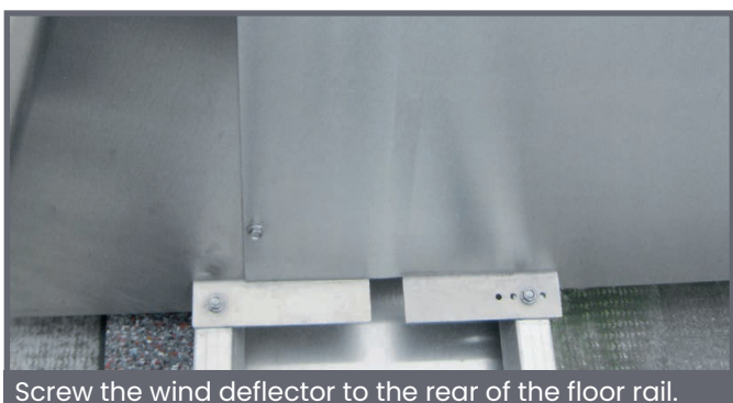
Screw on the spoiler at the front and rear using self-tapping screws
