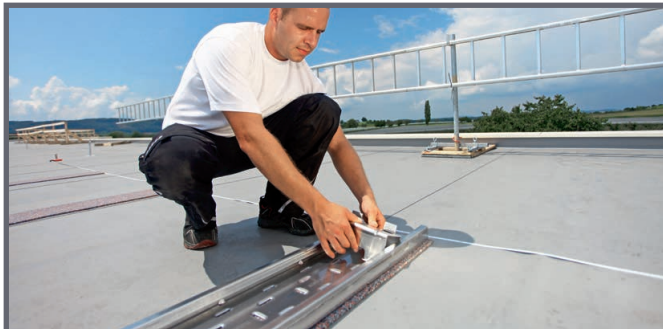
Inserting the front (short) module support
