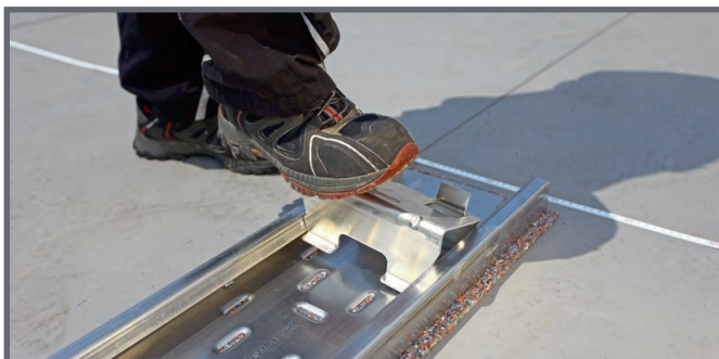
Clicking in the front module support
