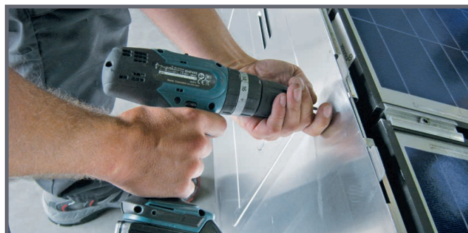
Screw the top and bottom wind deflectors together.
