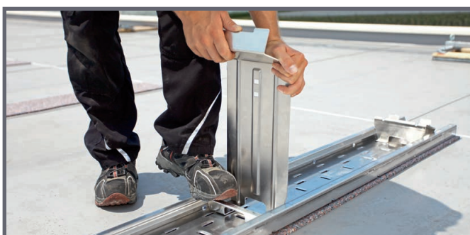
Clicking in the upper (high) module support
