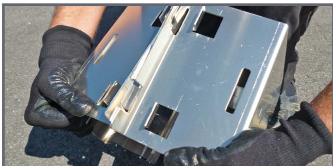
Interlocking the two rear module supports
