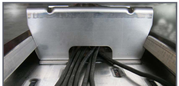
Floor rail used as a cable duct for the string cables
