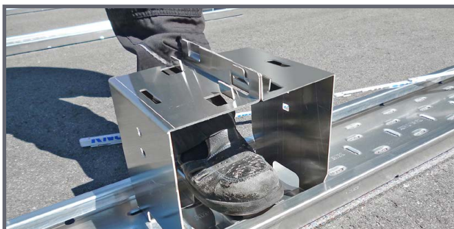
Clicking in the module supports
