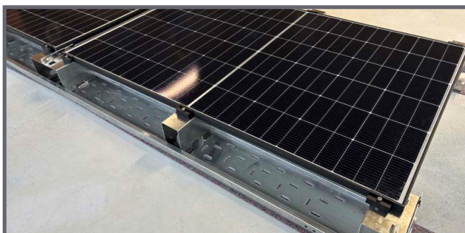
Fully assembled first row of modules
